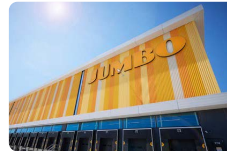
Mechanised distribution centre in Nieuwegein.
